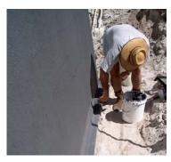
When termite proofing and water proofing in these situations, TERM-seal is a two in one application.
