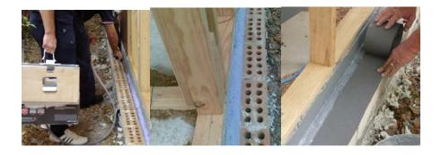
The three stages of installing **TERM-seal Urafen (0.2% Bifenthrin as active constituent)** as a termite cavity protection system
