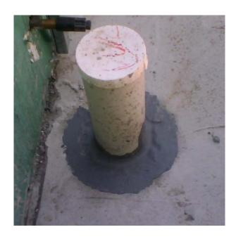
When a slab penetration has not been protected during the pour stage, TERM-seal Sealant Passive or TERM-seal Sealant Ative can be installed
